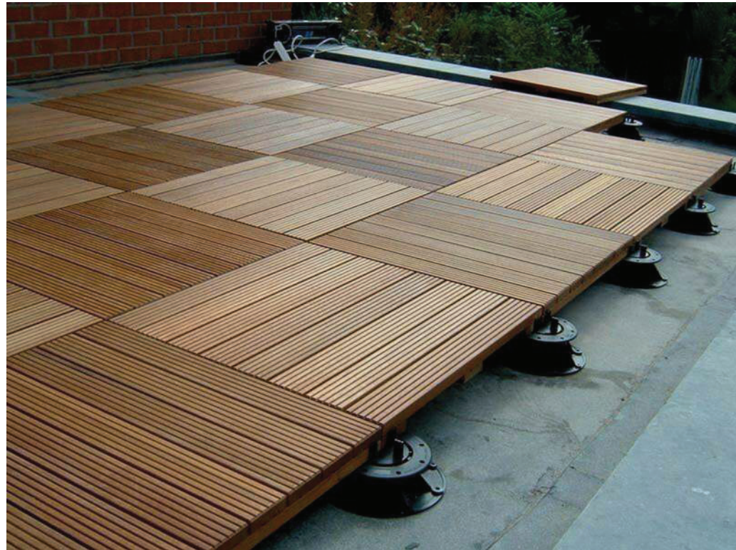
WOOD DECKING ON PEDESTALS such as Bison bamboo tiles
