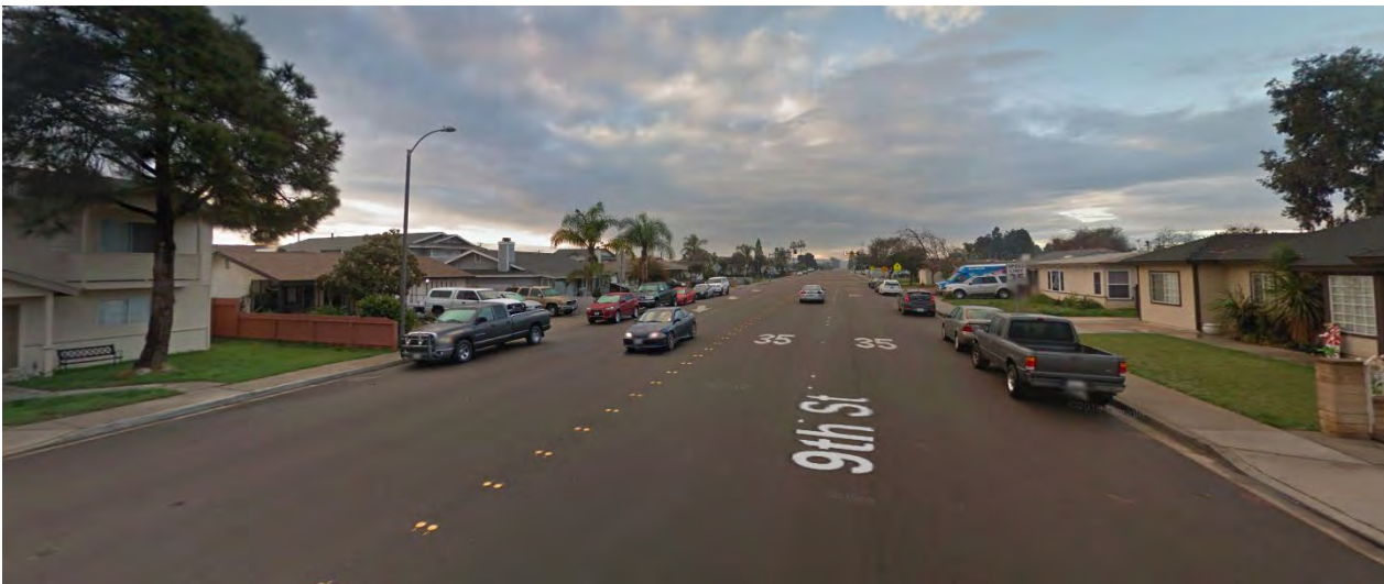
Figure 31. Existing 9 th Street Conditions
