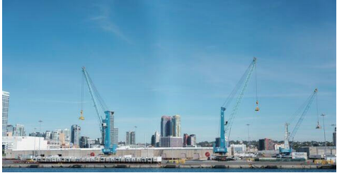
Tenth Avenue Marine Terminal Redevelopment ( /projects/tenth-avenue-marine-terminal-redevelopment )
