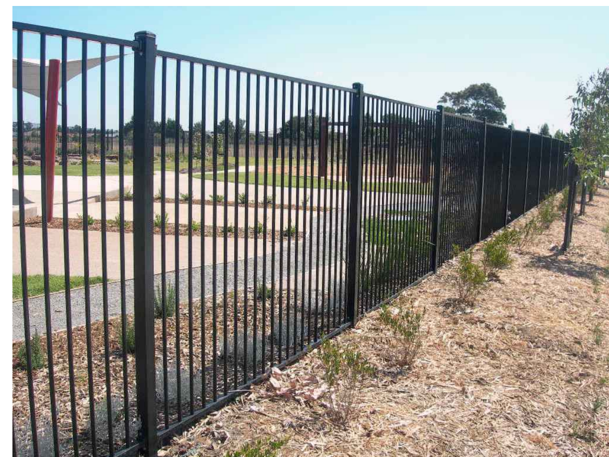
Decorative Wrought Iron Fence 4' high in the front setback, 6' high along the alley
