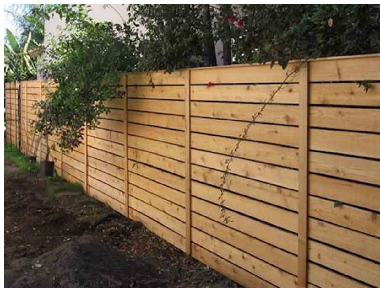
Wood Privacy Fence 4' high in the front setback, 6' high along the driveway
