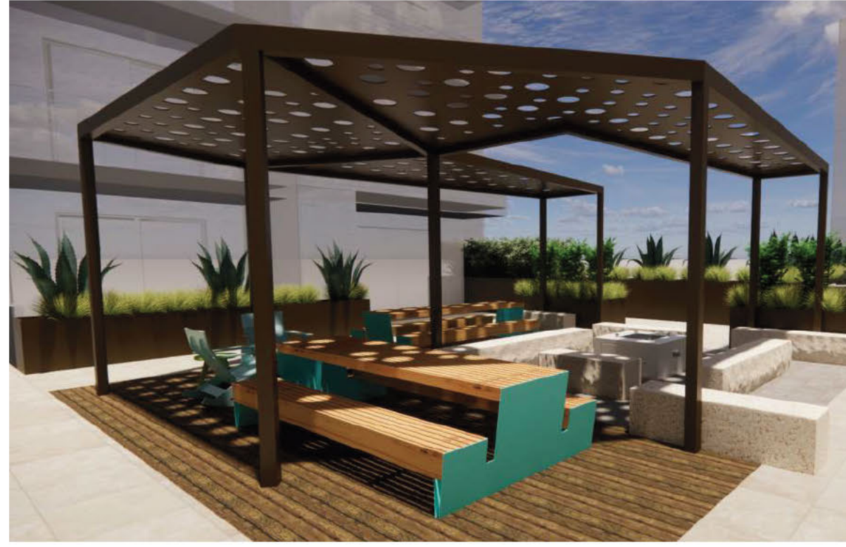
SHADE STRUCTURE steel frame, perforated metal canopy
